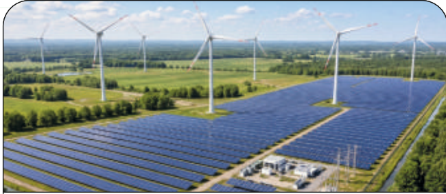
Hybrid Power Plant
